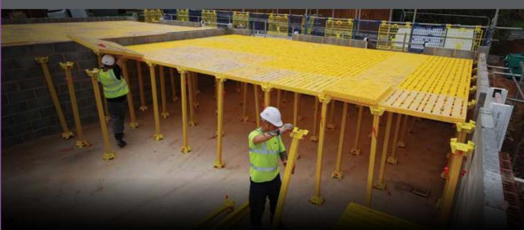
TRAD Safety Decking is an innovative, market leading fall prevention solution for traditional build projects, predominantly house building. The system vastly improves safety compared to traditional methods such as airbags, and is significantly quicker to erect and dismantle compared to a bird cage scaffold.
