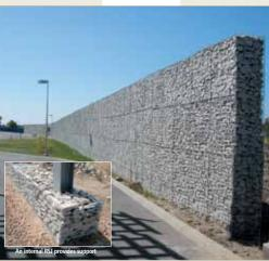
! A free standing, internally supported perimeter wall provides strength and durability for the new Gillette factory in Lodz, central Poland. Constructed 2005.
