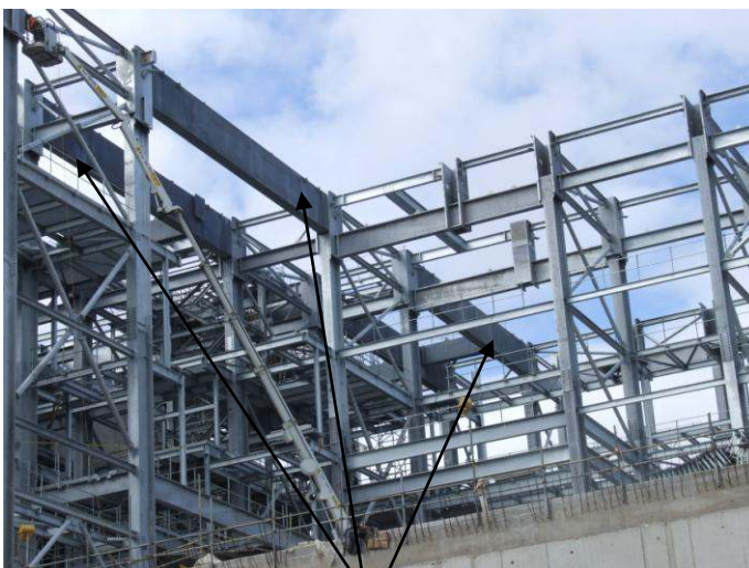
Zingaised beams in position
