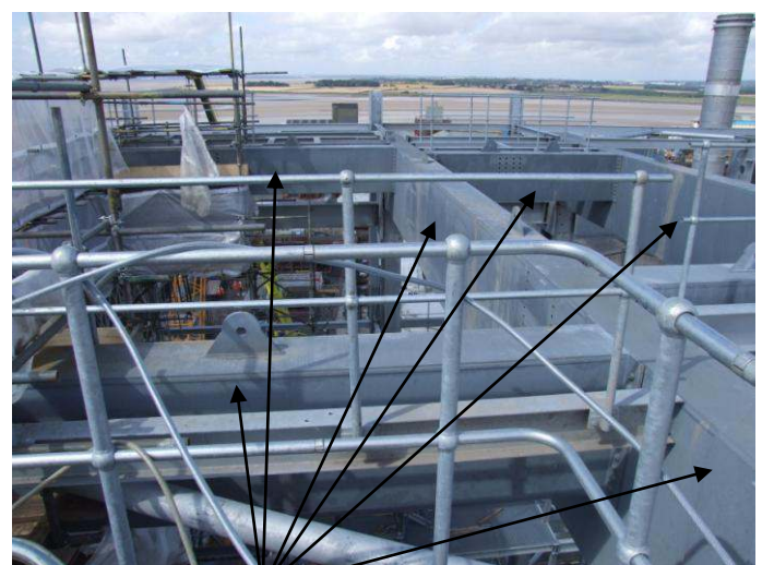
Zinganised beams on the top of the structure
