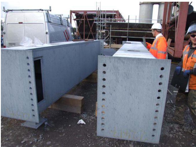
Checking the zinc-thickness on the zinganised beams
