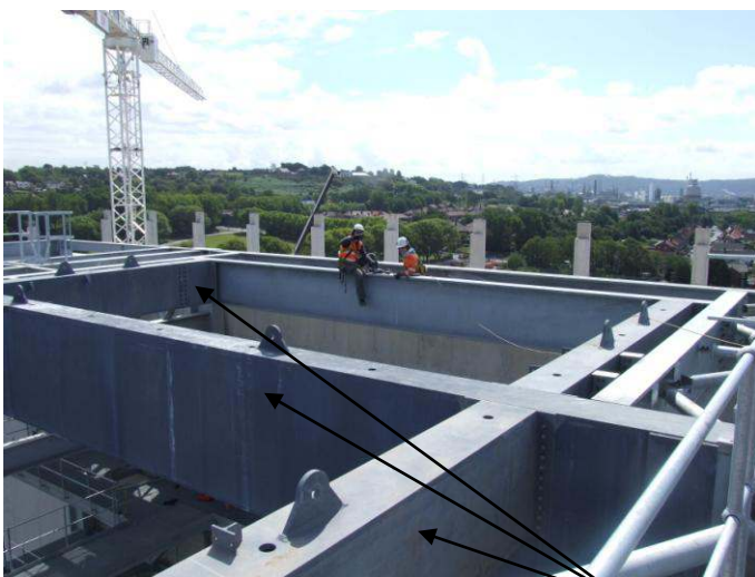
Zinganised beams on the top of the structure
