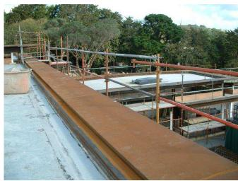
Above: The steelwork of the top edging-panels around the entire roof
