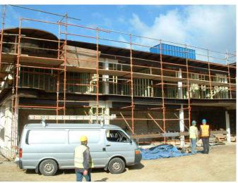
Above: A view showing the H-beams that were hidden by brickwork
